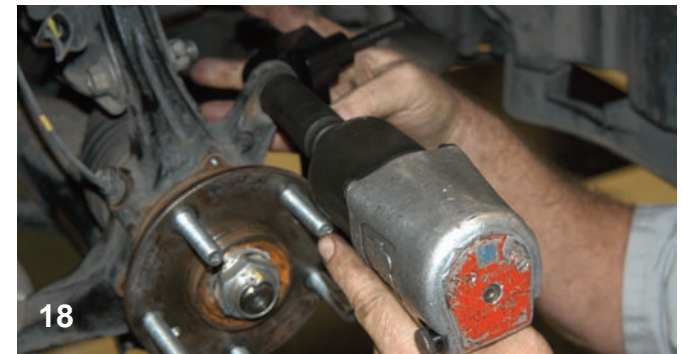
18 After the bracket bolts were started, they were tightened with an impact gun followed by tightening them again to 65 ft-lbs with a torque wrench.
