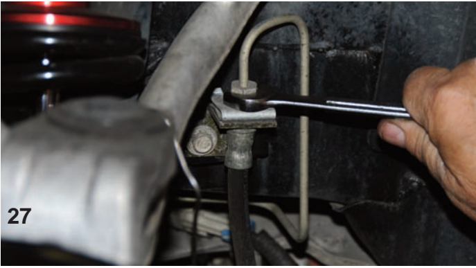
Using a line wrench, the hard line to flex line connection was broken loose prior to removal.
