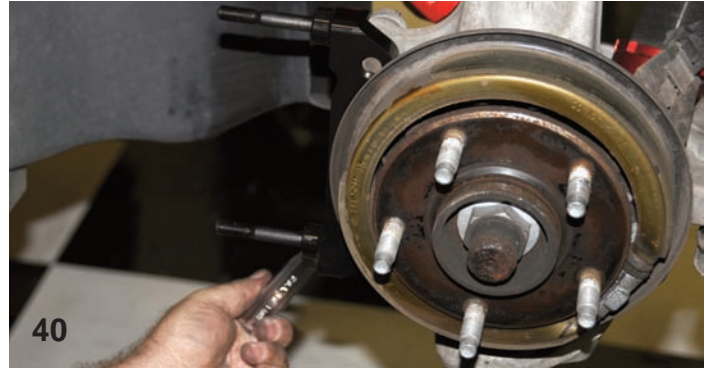
40 The bolts were screwed into the bracket and then they were tightened with a small socket wrench. Here the bottom bolt is being tightened.
