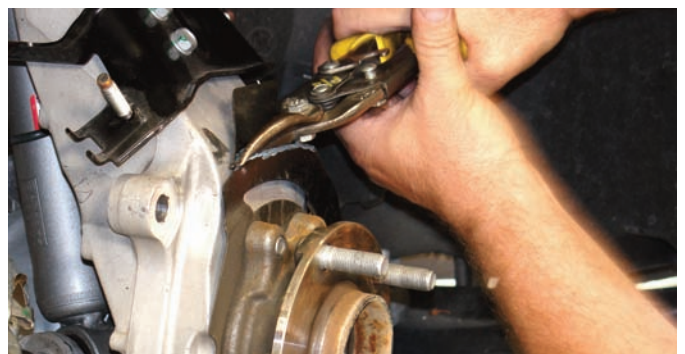
The metal can be removed with a three-inch cutoff wheel or with hand shears. Tony selected the hand shears because it is faster for a small operation like this.
