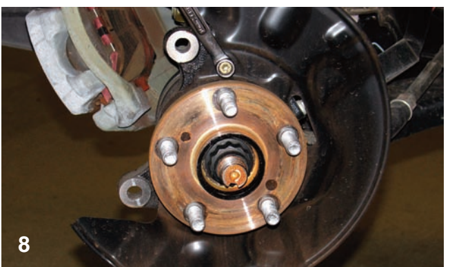
8 The dust shield will not be used, so the securing bolts were disconnected in preparation for removal.
