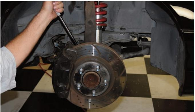
Using a large breaker bar and the appropriate size socket, the caliper bolts were broken loose.
