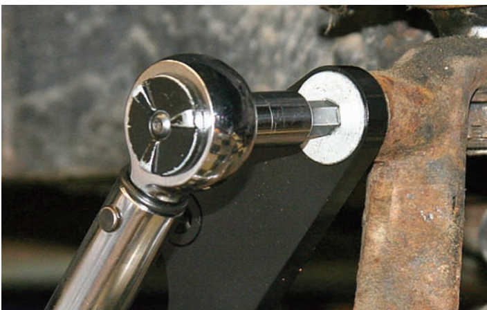
The upper Allen bolt was tightened to 77 ft-lbs using a foot-pound torque wrench and an Allen head socket.
